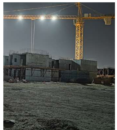
Baghdad Bodour / IRAQ 1.000 Double Storey Villas
