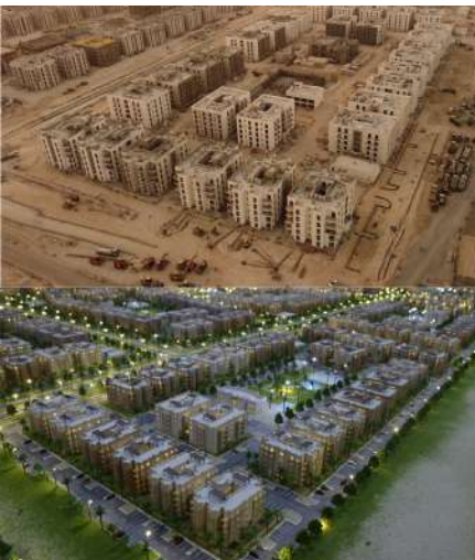
Doha / QATAR 6.780 Apartment
