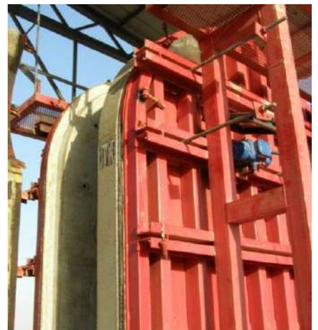
Al Anbar Stadium / IRAQ Retaining Wall
